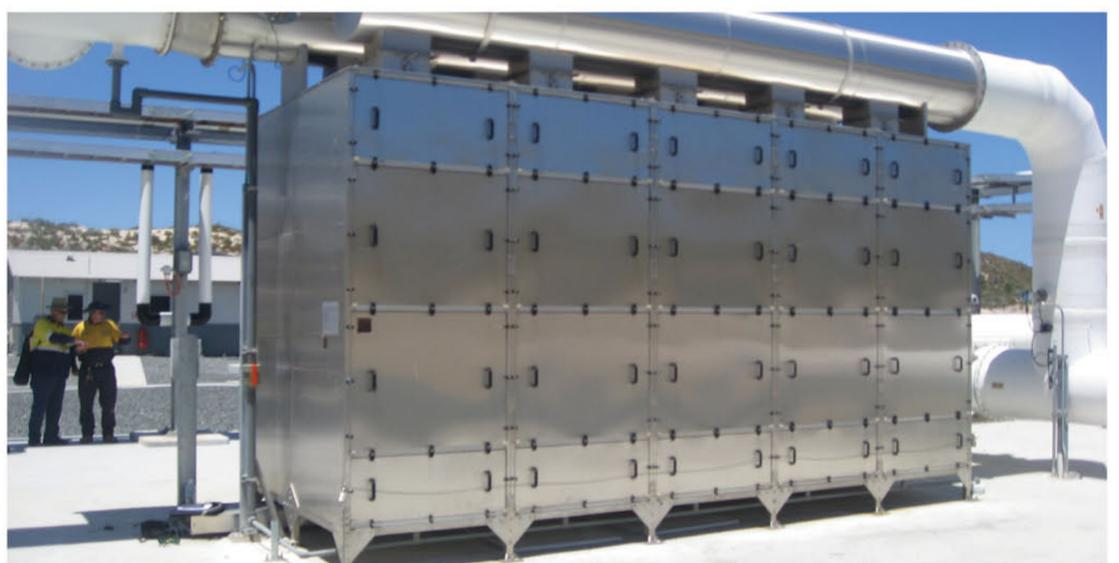
The Photoionisation process produces strong oxidizing agents via UV-light ionisation and these agents oxidize the odorous substances in the presence of catalysts leaving an odour free discharge.
