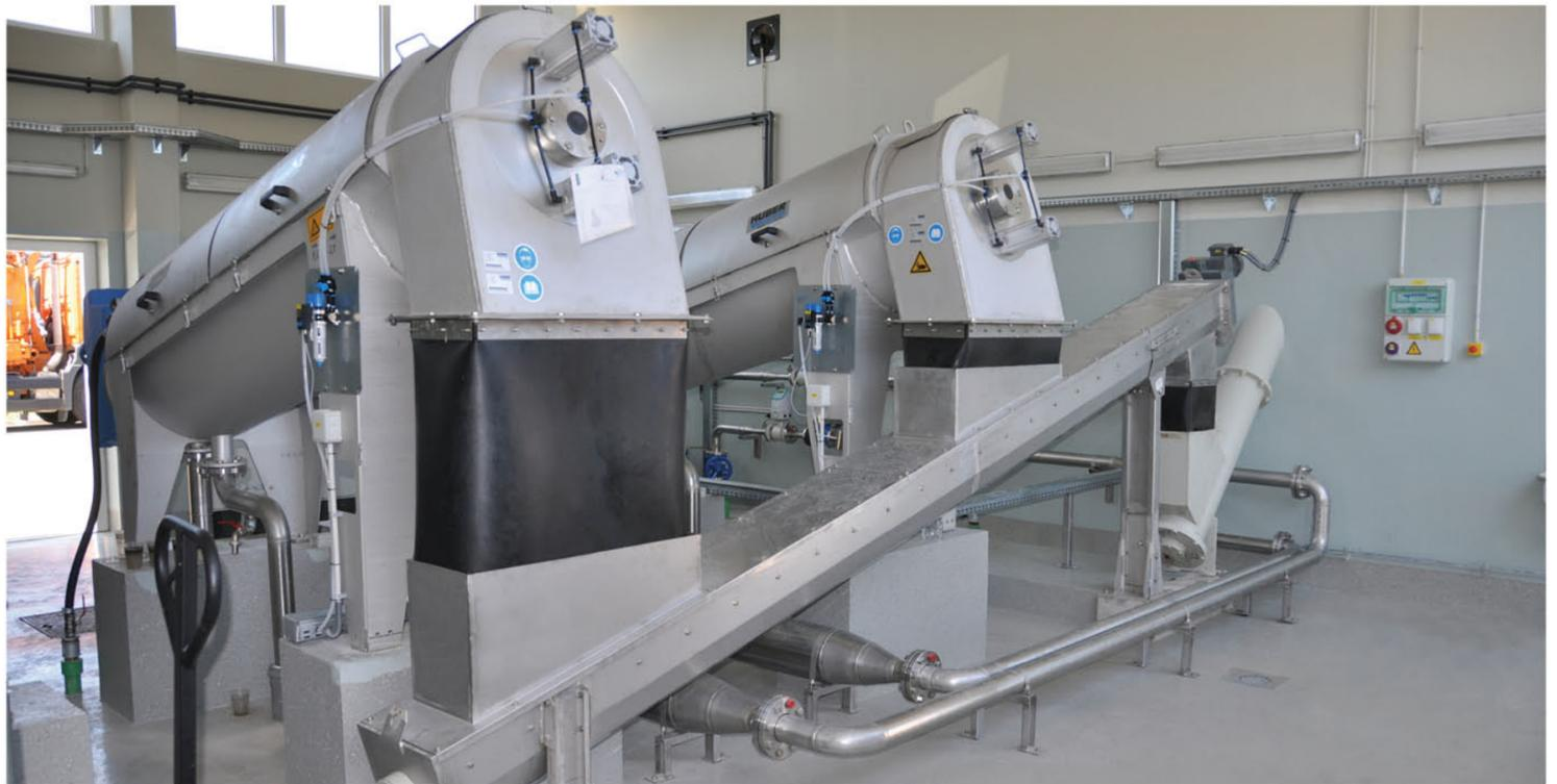
A HUBER screw press dewatering combined primary and secondary sludge at an industrial plant in Sydney
