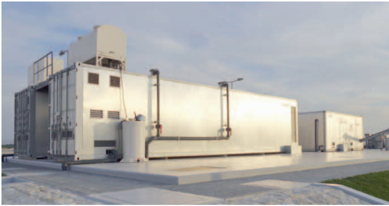
MENA Water ultramodern wastewater technology – ideal for decentralised wastewater treatment
