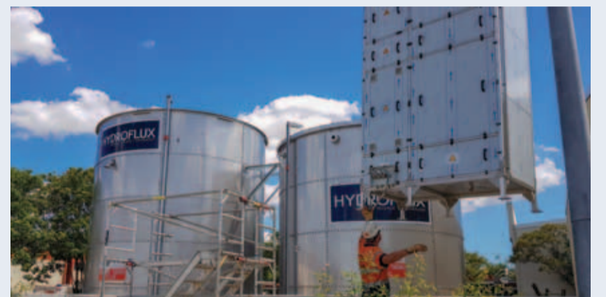
3500m 3 /per hour Neutralox system being delivered to a food processing plant
