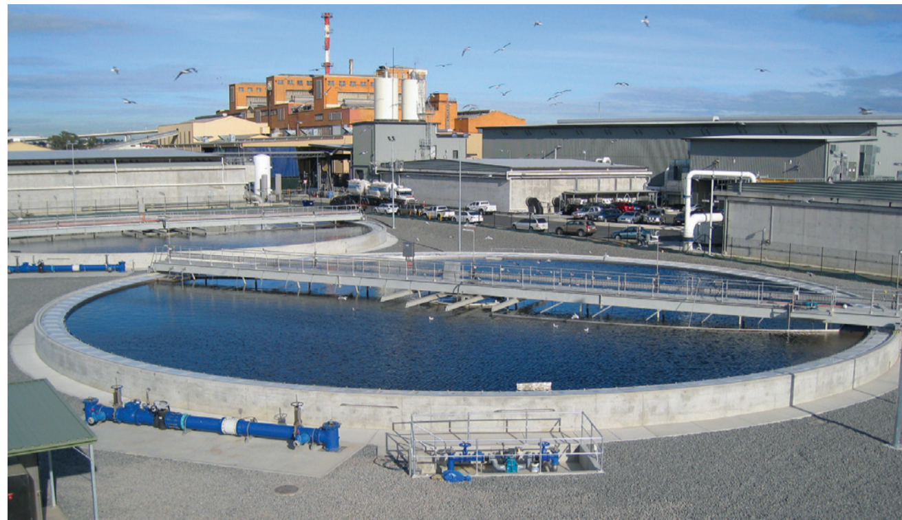
A Hydroflux Epco 45 m diameter LogMAX® clarifier installed at Gibson Island Sewage Treatment Plant
