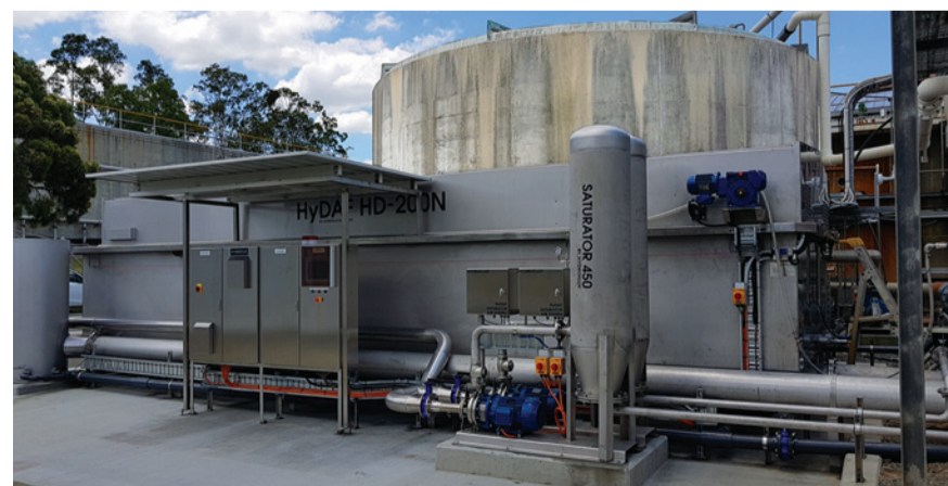
A Hydroflux HD200 HyDAF System at a Brewery Specifically Designed for Removal of Anaerobic Biomass from Wastewater
