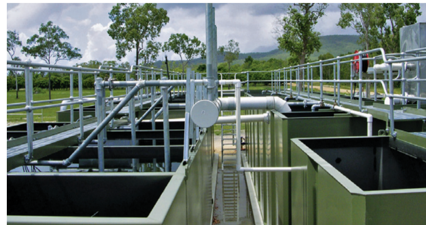
A Hydroflux EpcO RoadTrain™ packaged STP at Pt Hinchinbrook Resort
