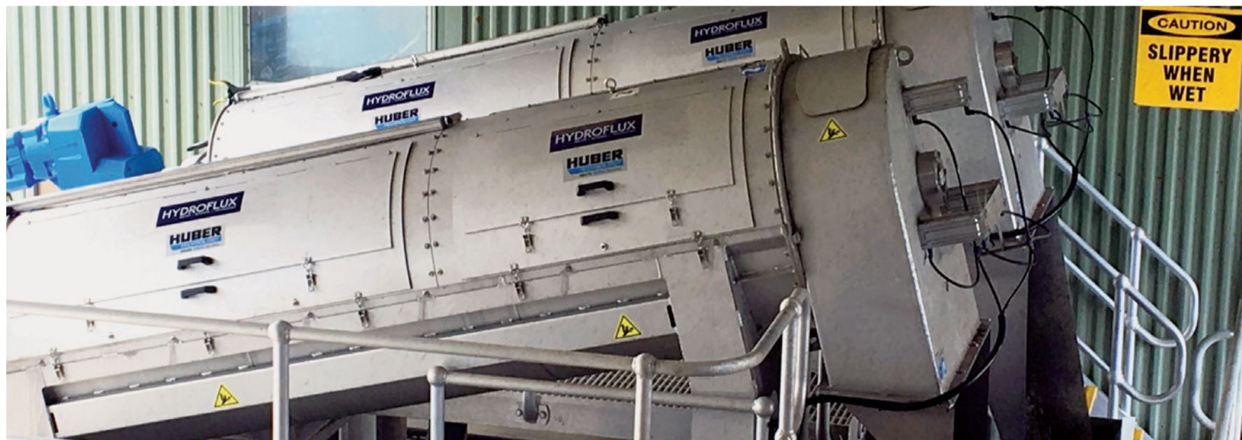
Dual screw presses and conveyor installed at Bribie Island WWTP
