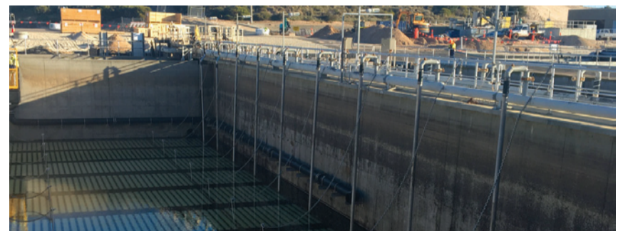
High efficiency AEROSTRIP™ diffusers at Bunbury WWTP
