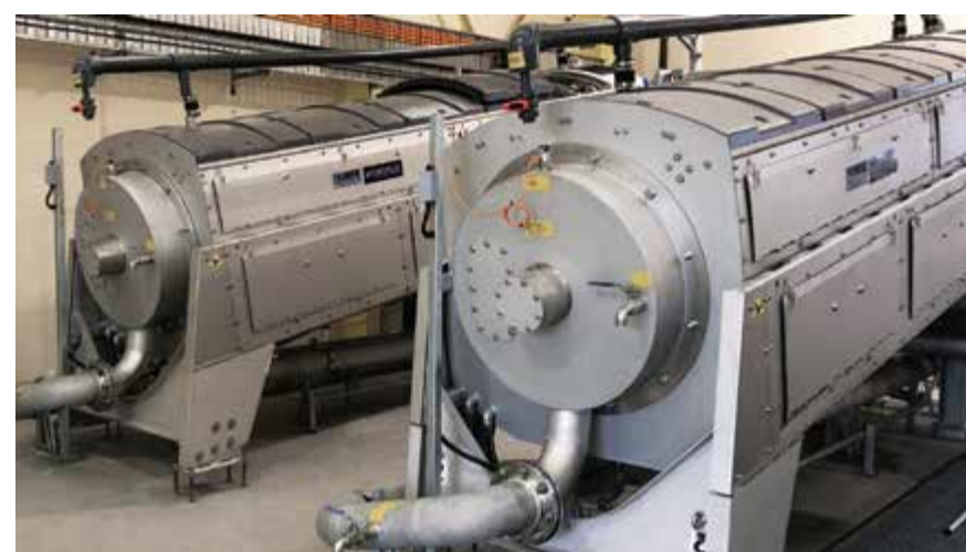
Two Huber Q800 screw presses installed at Ti Tree Bend STP, TAS.
