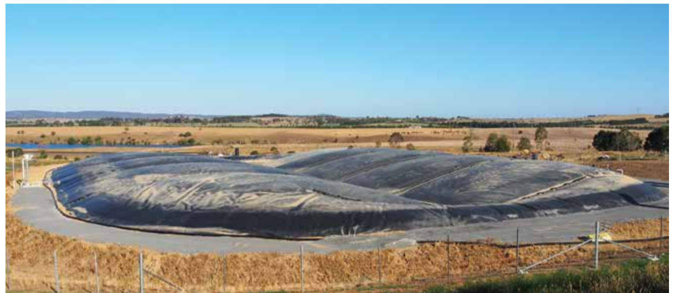
Anaerobic lagoons provide a very effective means of wastewater treatment.
