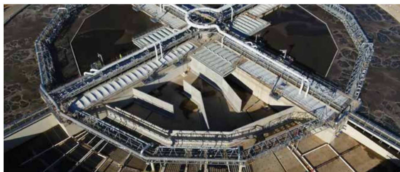
An aerial view of an AEROSTRIP® during the installation process
