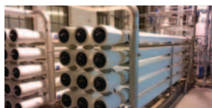
The key processes for Flootech demineralized water treatment are FlooIX™ Ion exchanger, FlooRO™ Reverse osmosis and FlooMB™ Mixed Bed ion exchanger.
